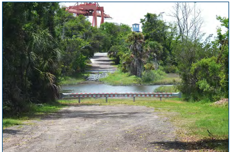
Looking north across the Escambia Street road bed and Escambia Slough, after removal of the culvert. A container crane and the widow's walk of the Port Authority's "Blue House" are visible in the background.
