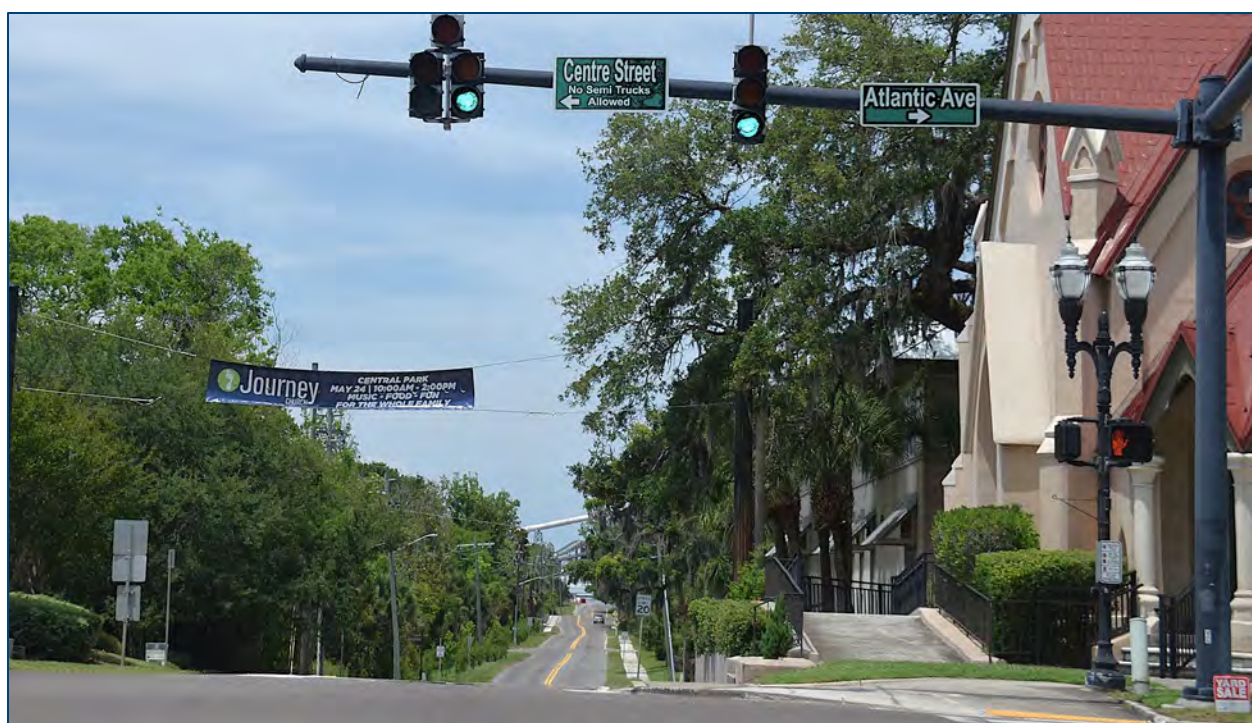
Below: Looking north at Centre Street/Atlantic Avenue, the turning radii at the northeast corner is constrained. Also, the street name plaque indicates no trucks may turn onto Centre Street.
