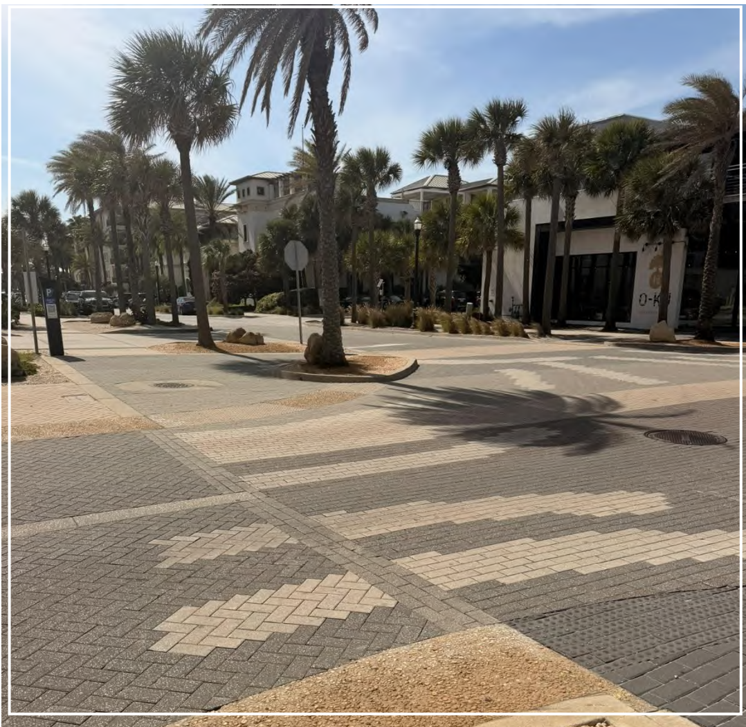
Pedestrian facilities on First Street. Source: Project Team.
