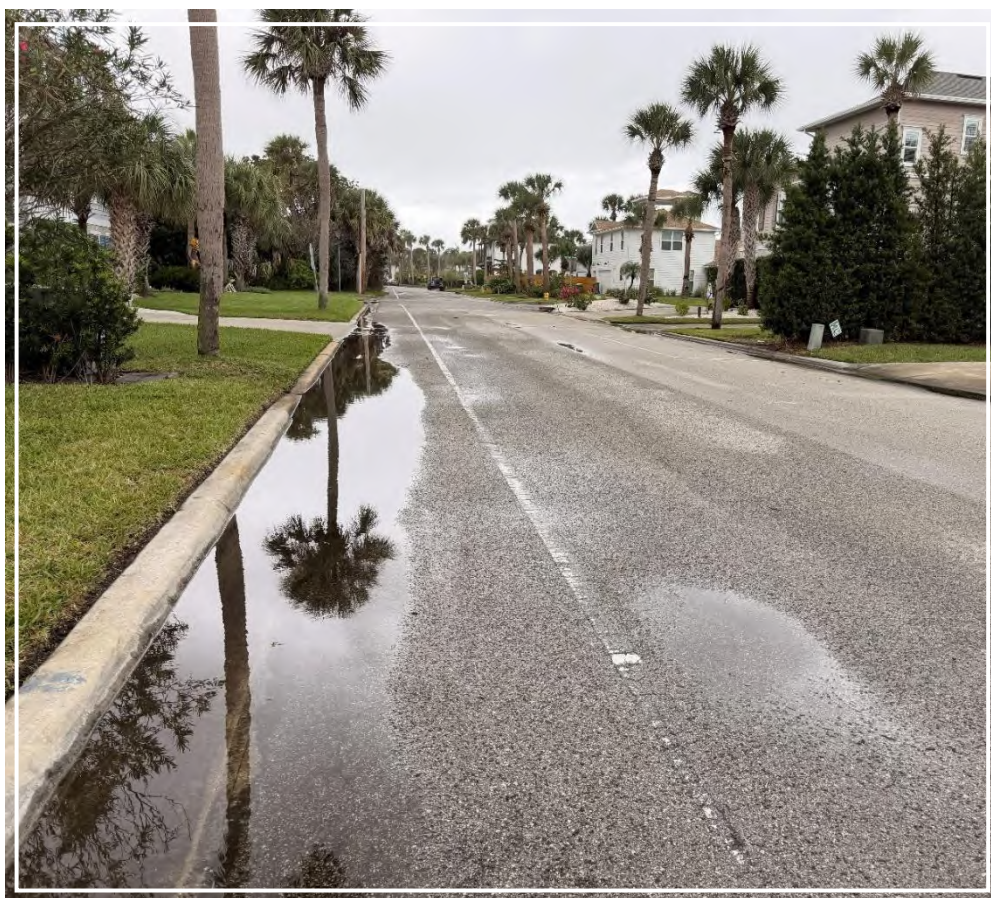
Standing water along First Street after a storm. Source: Project Team.
