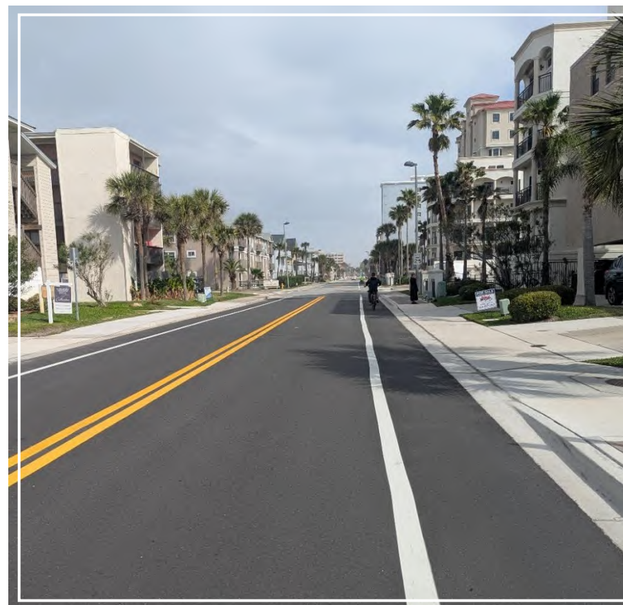
Streetview of CA-2. Project Team.
