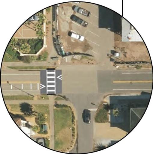
Add raised crosswalk
