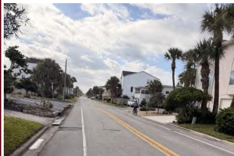
Roadway edge in South Jacksonville Beach.
