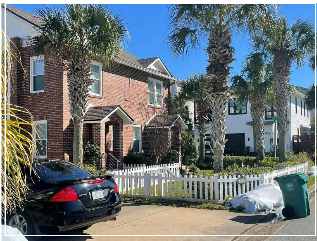
Existing multi-family residential along First Street. Source: Project Team.
