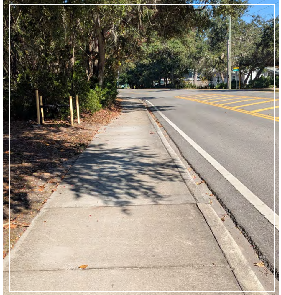
Curb and gutter drainage on Citrona Drive. Source: Project Team.
