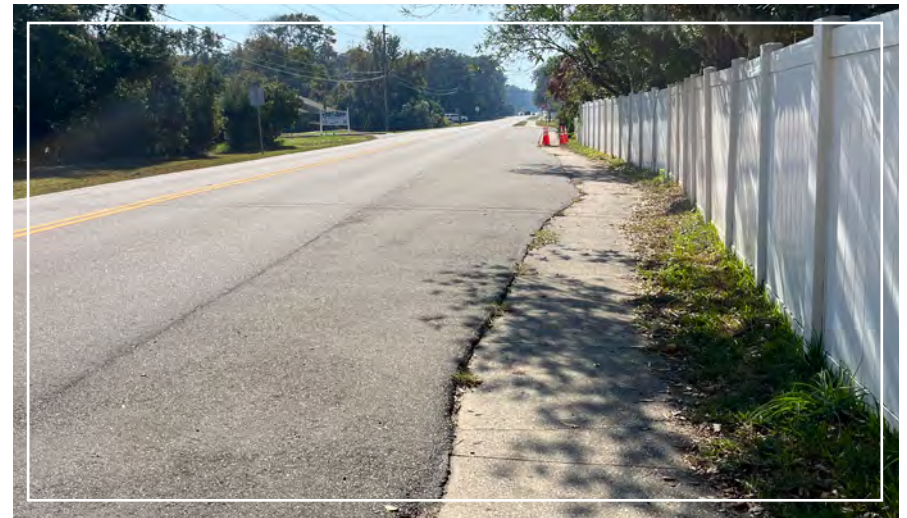
Constrained right-of-way Citrona Drive. Source: Project Team.
