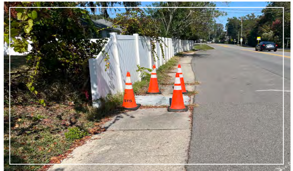
Sidewalk adjacent to traffic on Citrona Drive. Source: Project Team.
