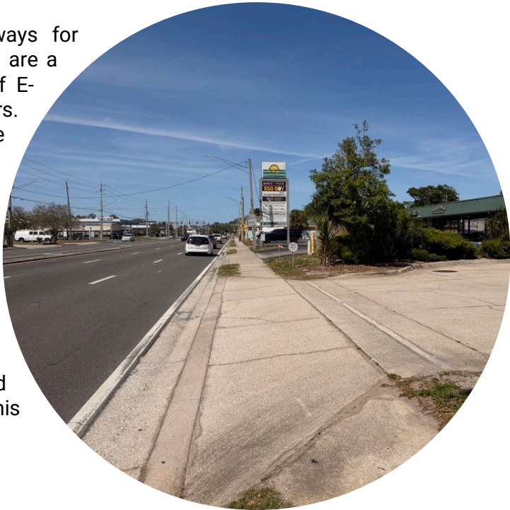
Photo 4. Driveways on Mayport Road (A1A) Facing North
