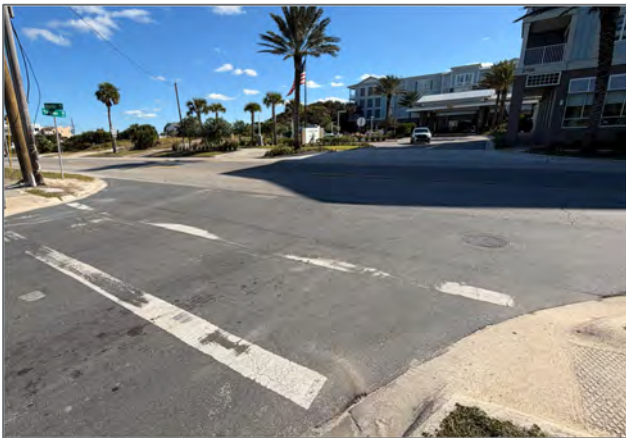
Faded crosswalk markings and lack of detectable warnings at curb ramps on Tarpon Avenue, looking south.
