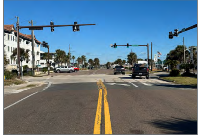
Existing pavement and markings conditions on S Fletcher Avenue, looking north.
