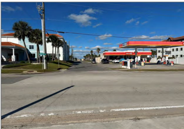
Existing pavement conditions on Tarpon St near Circle K, looking north.
