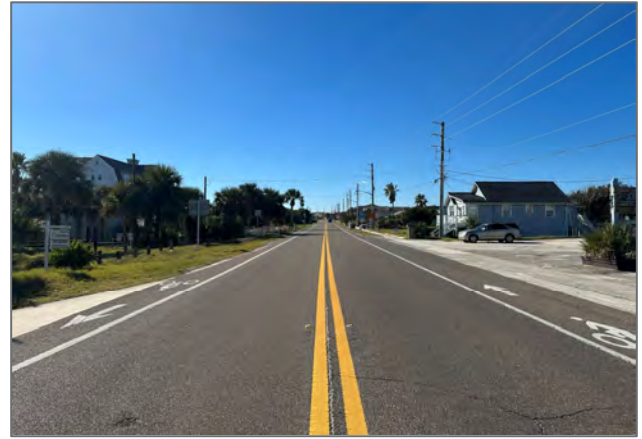
Existing travel lanes and bike lanes on S Fletcher Avenue, looking south.
