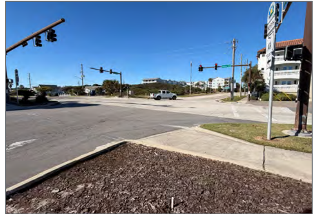
East leg crosswalk is faded, and the north leg crosswalk is lacking ADA curb ramp.
